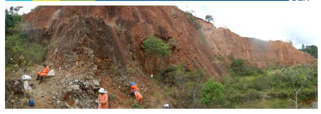
Figure 9-2: Channel Sampling Program at the Cava Do Bezero Open Pit
