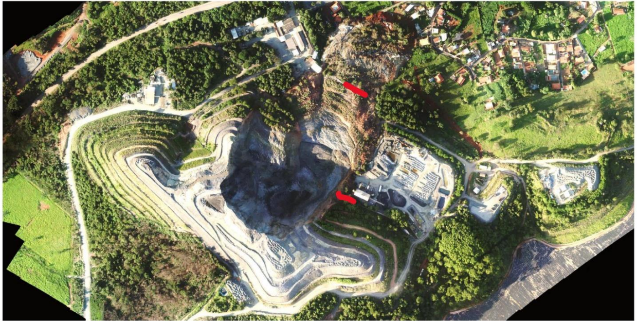
Figure 2: Immediate aftermath of the Satinoco tailings pile slump.
